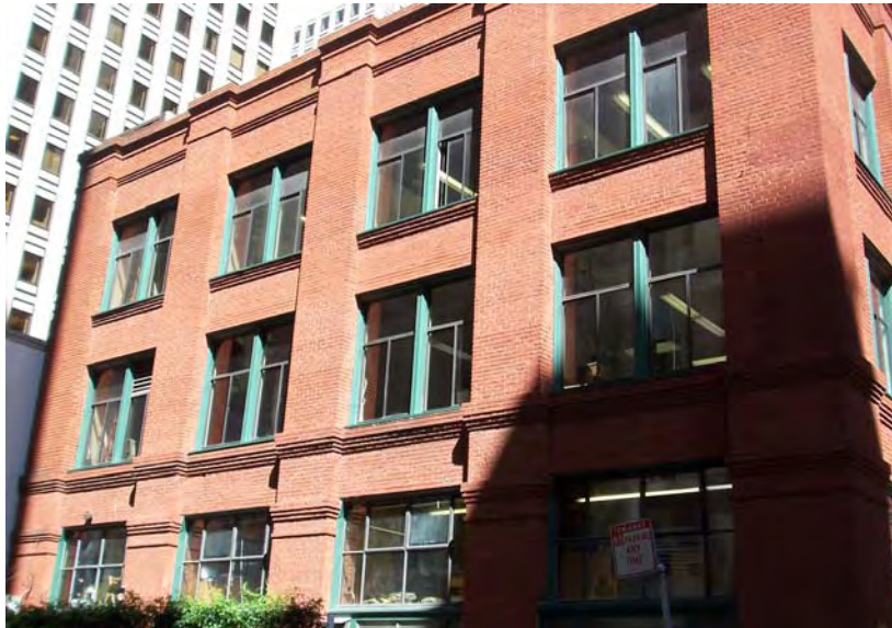
Figure 38. Warring-Wilkinson Building, 96 Jessie Street, 2007 Source: KVP Consulting
