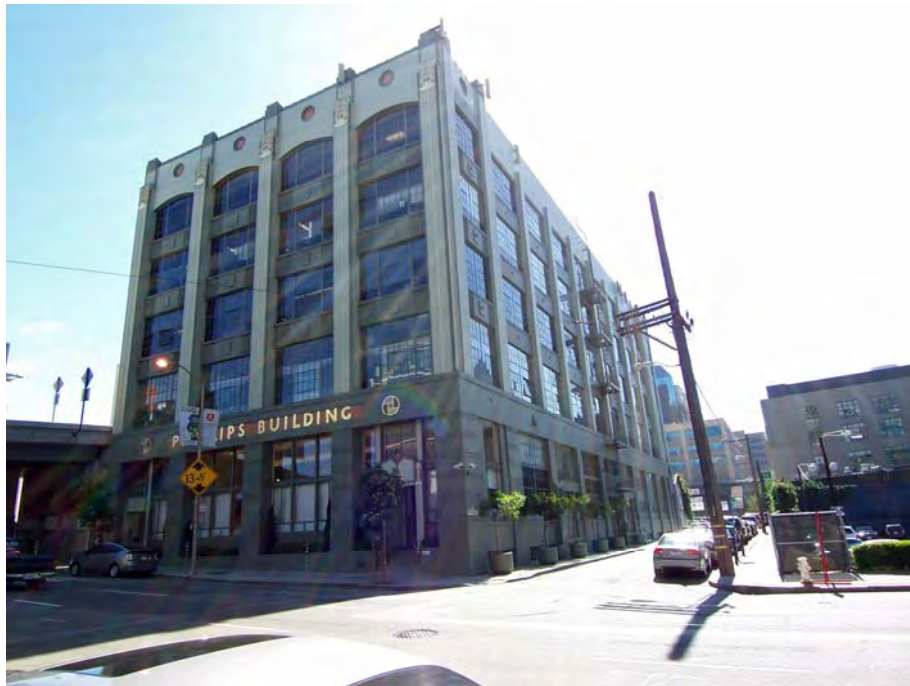
Figure 37. Philips Van Orden Building, 234 1 st Street, 2007 Source: KVP Consulting
