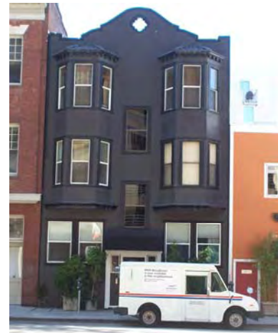
Figure 22. 568 Folsom Street Source: KVP Consulting
