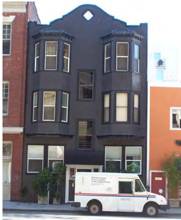
Figure 33. 568 Folsom Street, 2007 Source: KVP Consulting
