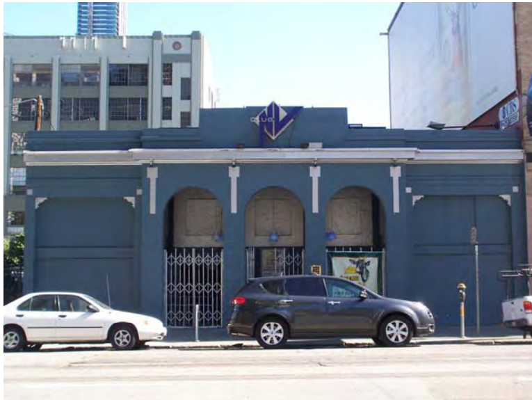
Figure 34. Louis Lurie Building, 525 Howard Street, 2007 Source: KVP Consulting
