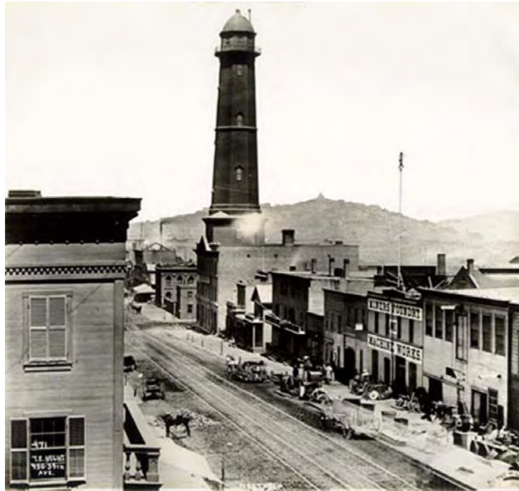
Figure 13. Selby Shot Tower, 1 st and Howard Streets, 1868 Source: San Francisco Public Library
