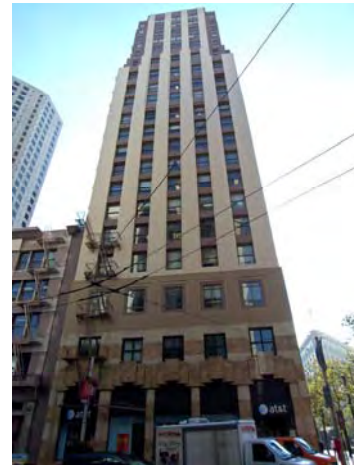
Figure 24. Central Tower Source: KVP Consulting
