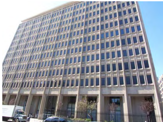
Figure 29. 666 Folsom Street, 2007 Source: KVP Consulting
