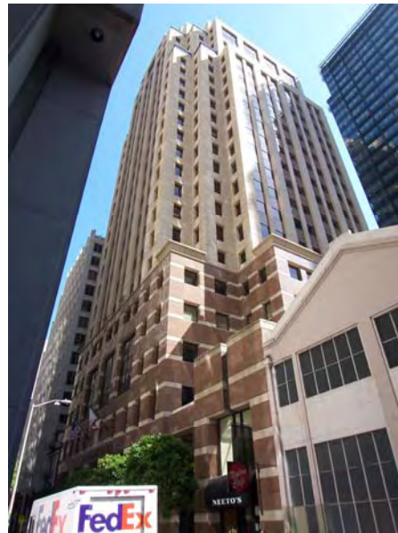
Figure 31. 71 Stevenson Street, 2007 Source: KVP Consulting
